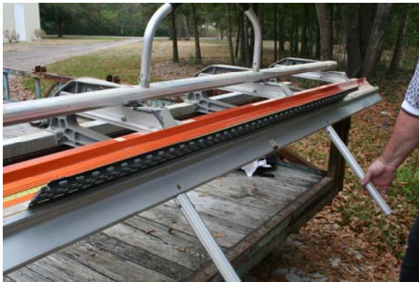
Field forming for fascia mount applications using a small sheet metal hand brake
