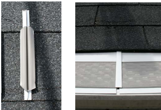
H-Splice Butt Joint
