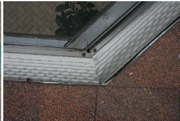
Field forming for fascia mount applications using a small sheet metal hand brake
