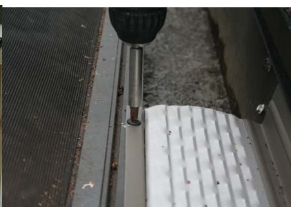
Secure in place to the gutter lip
